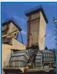
Centrifugal mine fans are designed for drawing air of temperature up to 60°C, out of underground mines.
